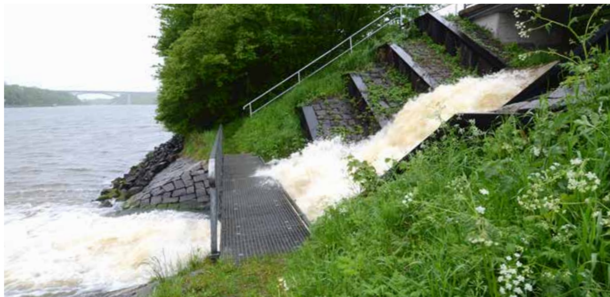
Drainage sluice at Projensdorf
