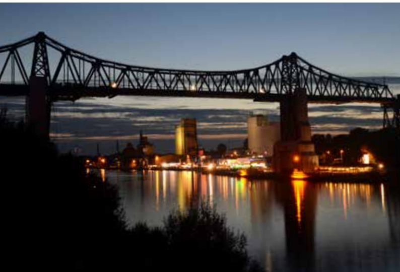
Rendsburg high-level railway bridge
