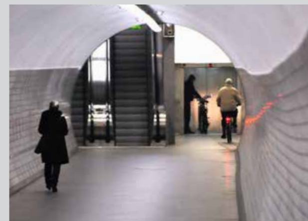
Sehestedt ferry crossing Rendsburg pedestrian tunnel
