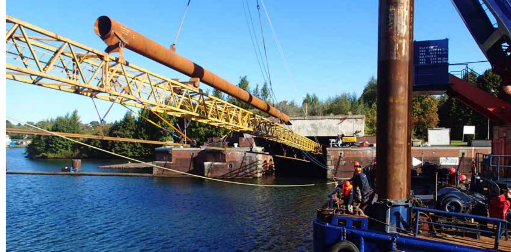
Replacing the rails in the large chambers at Kiel-Holtenau
