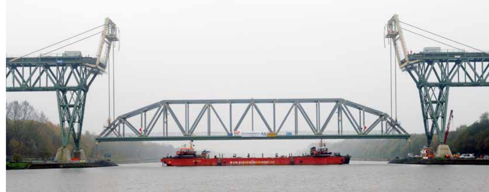
Inserting the middle section of the high-level railway bridge at Hochdonn.
